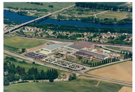
Pont à Mousson (France) is the headquarters of DR FISCHER Europe S.A.S., the production center of infrared halogen lamps, UV lamps, high-voltage lamps, halogen and incandescent lamps.
