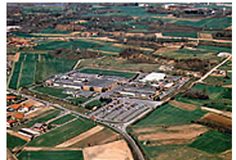
DR FISCHER Italy s.r.l. produces special lamps for the domestic field at the Alpignano (Italy) location
